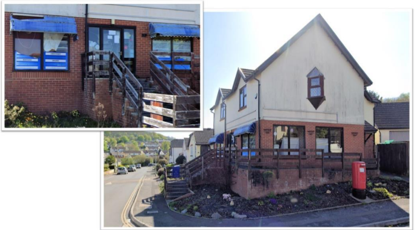
FIGURE 2 – IMAGE FROM GOOGLE STREETVIEW APRIL 2022 © GOOGLE
